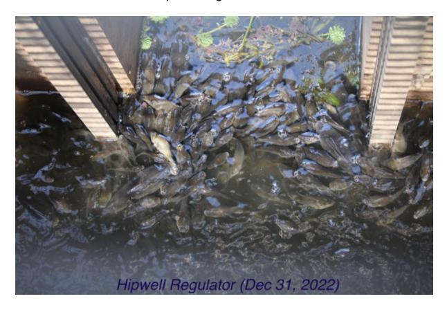
At 7:00am and 7:00pm the exit and entry gates on the fish lock operated to allow the fish (carp) on the forest side of the regulator to enter Gunbower Creek.
