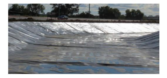
Above: Remediated channel lined with HDP. Fresh water Turtles cannot exit plastic lined channels.
