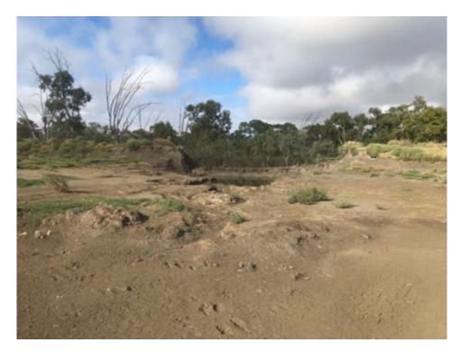
One of the many flood bank breaches that needs fixing.
