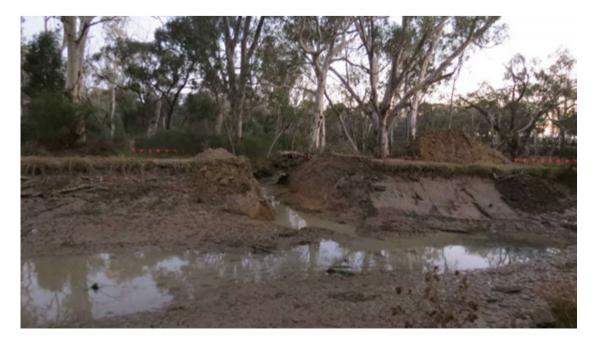
Above: Channel 2/4/1 -cut made by excavator to drain water from the channel for works to begin.
