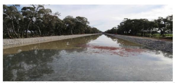
Above: Channel 2/4/1 from the top-Clay lined, HDP lined, crushed rock and Rock wall finish. Works completed between May and August 2017.
