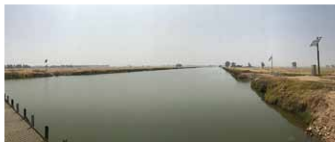
Mulwala Canal, December 2019. Photo commissioned by Berrigan Shire Council
