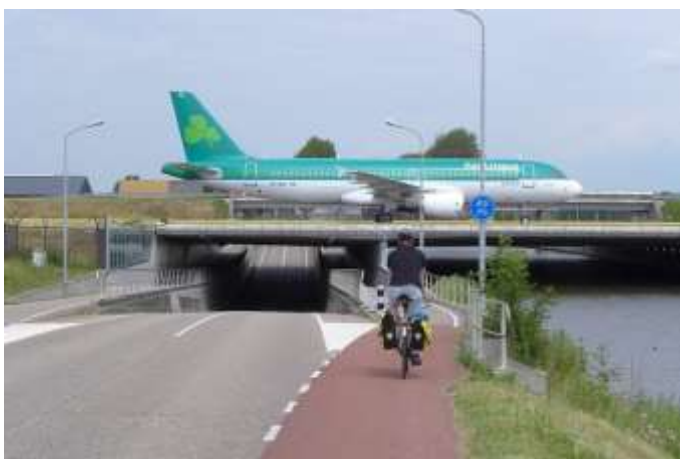
Underpass at Amsterdam Schiphol Airport with cycle and pedestrian facility.
