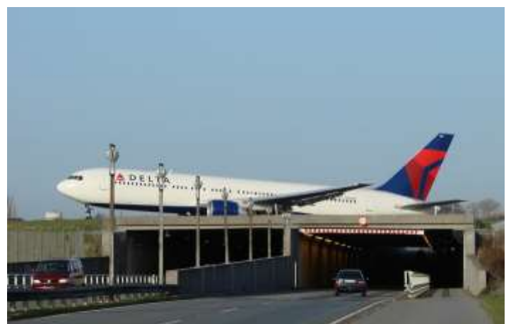
Taxiway underpass at Manchester Airport with a pedestrian pathway.
