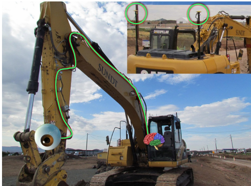
Image: Steve Jones/McGraw Hill: Driverless digger: Illustrating increased automation for site-works
