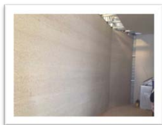
HEMP WALL ON LOCATION IN BALLAN
