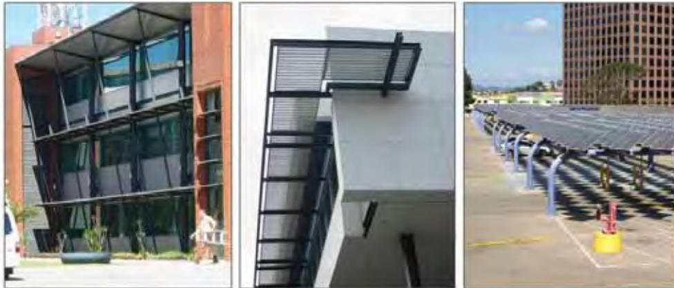
Examples of design solutions for reducing energy consumption through the use of passive shading controls, or through the use of active systems such as photo-voltaic arrays incorporated into car parking shade structures (which could be used to charge electric vehicles in the future).
