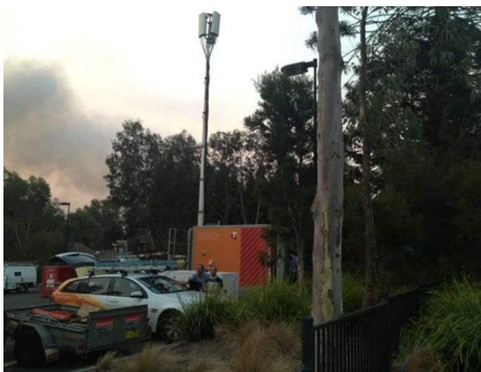
Figure 1: A COW at Winmalee shopping Centre, NSW to temporarily increase mobile network capacity during bushfires, October 2013
