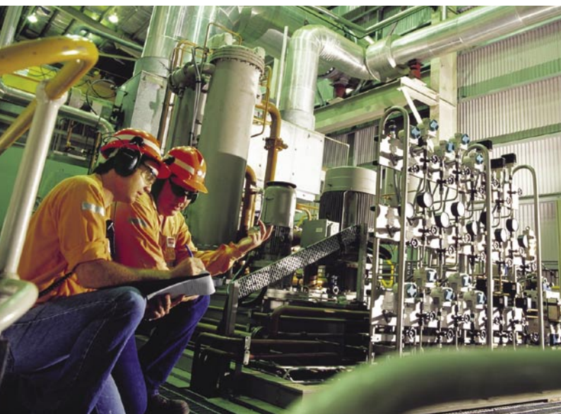
CSR Pioneer cogeneration mill using bagasse
