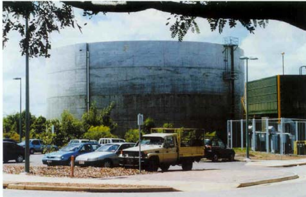
Thermal storage tank at the Casuarina Campus of the Northern Territory University
