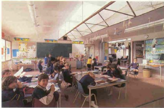
Interior of classroom showing light tunnel and baffles to reflect daylight.
