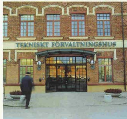
The retrofitted building in Eskilstuna.
