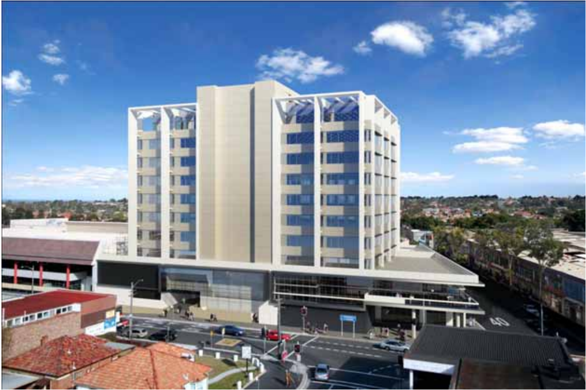
Artist impression of the 9-storey commercial office tower on club premises. The development application was approved by Bankstown Council on Tuesday December 8, 2009.
