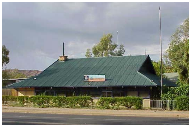
Former CWA Rooms, now the Bluegrass Restaurant, Alice Springs.
